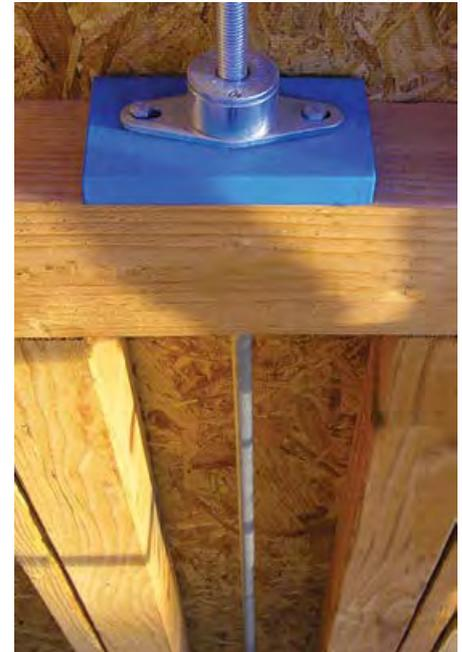
A continuous tie-down system with perpetual shrinkage compensation.
