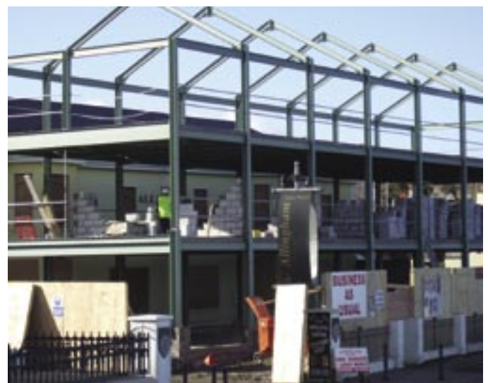
Steel and block construction, Clifton (seaside resort), Western Ireland.
