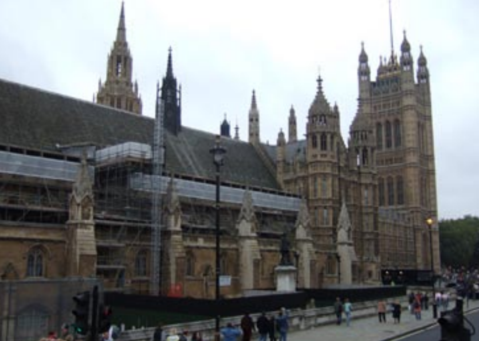
Repairs to Westminster Palace, London.
