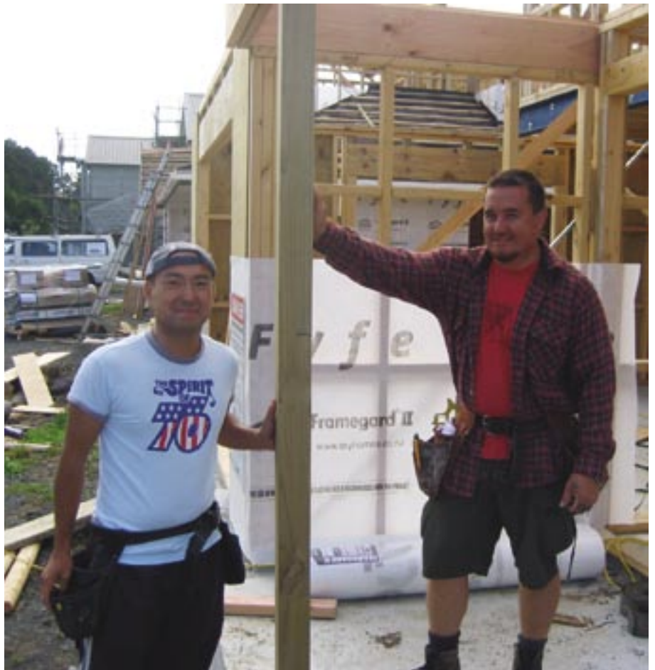
Kato Kazunao and builder Tangi Henry (contractor to Fyfe Homes).
