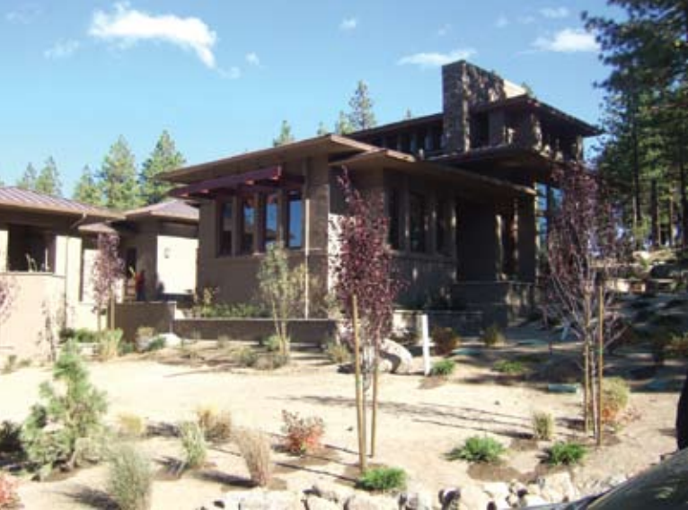
Million dollar home above Lake Tahoe (Washoe County) being built/inspected
