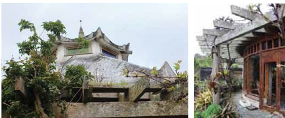
FIGURE 06 & 07: Correct use of passive design influences the thermal performance of an adobe house. Source: personal archive.
