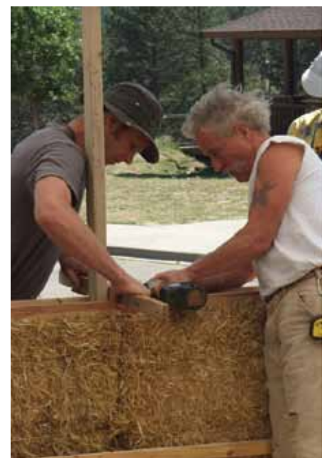
"Workshop participants taking part - Builders Andrew McCurdy from New Zealand and Tom Rijken from Holland building a straw bale wall"
