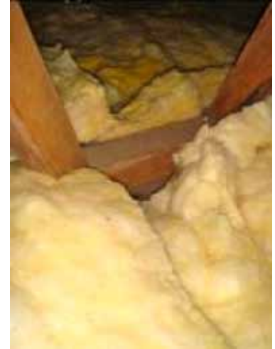
Badly laid insulation
