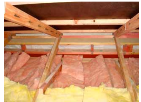
Badly laid insulation
