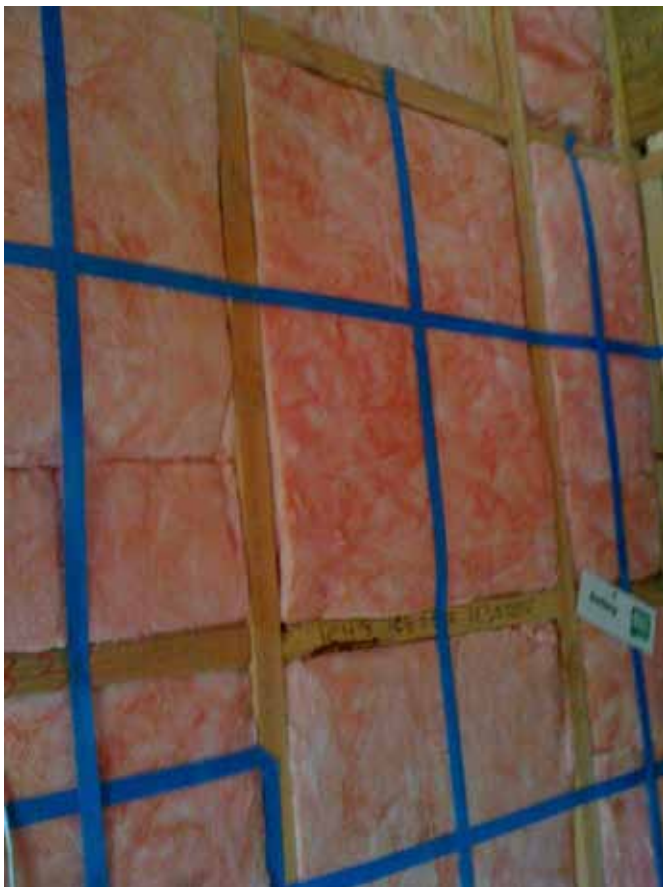
Strapping holds this insulation tightly in place
