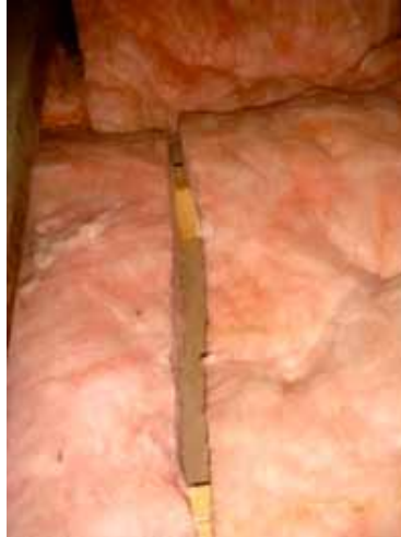
Gaps between blanket insulation laid in the ceiling will reduce the effectiveness considerably.
