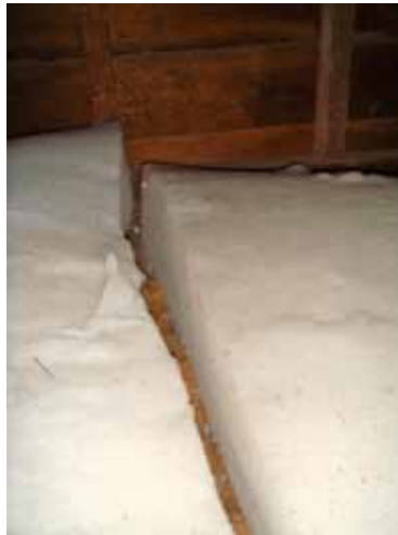
Gaps between blanket insulation laid in the ceiling will reduce the effectiveness considerably.
