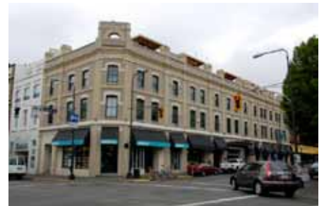
This Victoria CBD building has had penthouse suites added unobtrusively, set back from the road.
