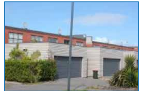
Houses in this development have their garages on the northern, sunny side, wasting the opportunity for solar gain.
