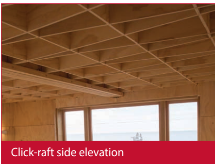
8.2 CLT ceiling panel assembly
