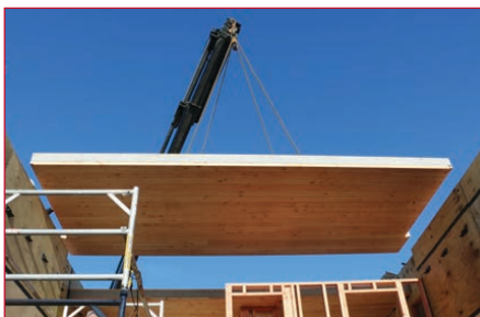
8.2 CLT ceiling panel assembly
